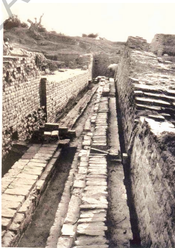
Fig. 20.8: Drainage system in a street in Mohenjodaro
